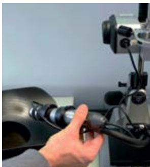
Visual quality control of the welding zone at the ELGEF Plus Branch Saddle Topload
